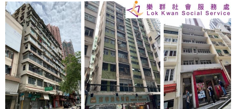
Existing Vacant Flats at Homantin / Central (86 Units)
