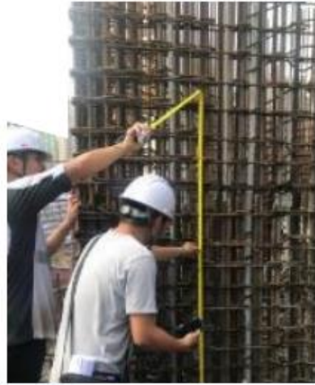
Site Work Inspection
