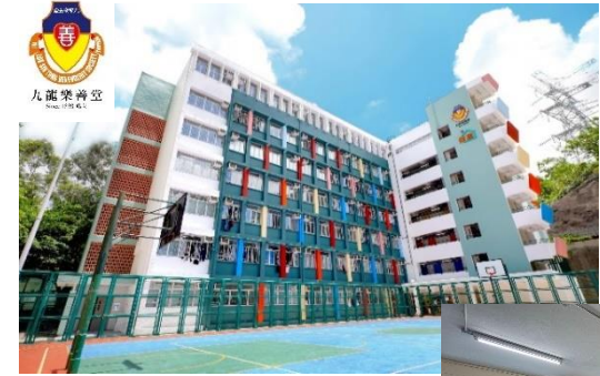
Former Tsuen Wan Lutheran School (145 Units)
