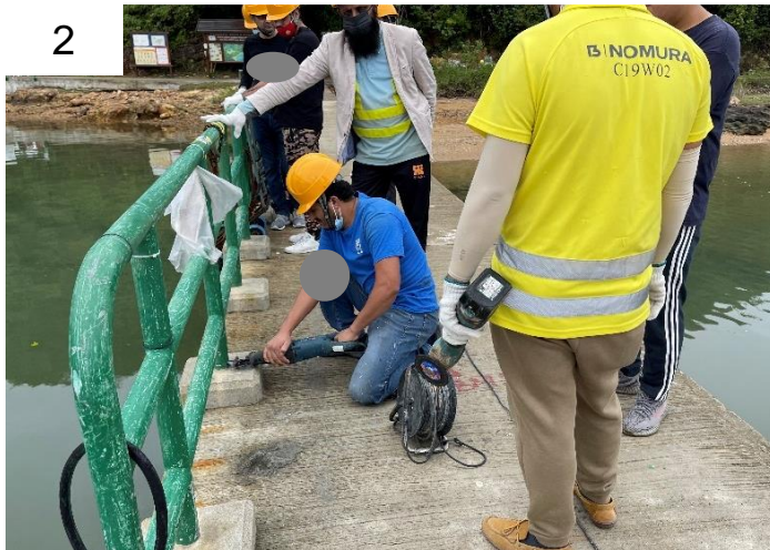
Removal of Barrier 拆除欄杆
