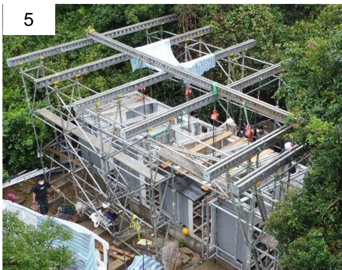
Lifting & Install 吊運安裝
