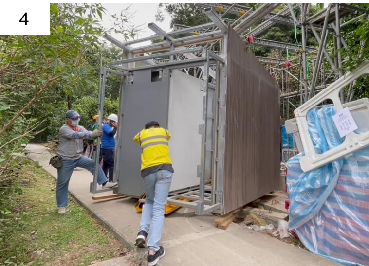
Scaffolding for Fixing 臨時棚架
